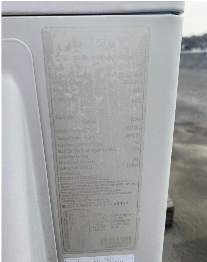
Figure 8 Nameplate of ductless split air conditioner.
