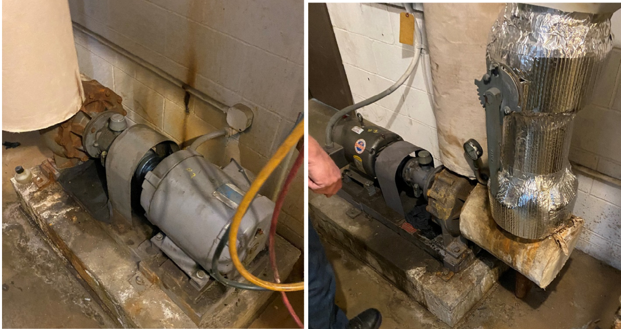
Figure 5 Chilled water pumps.
