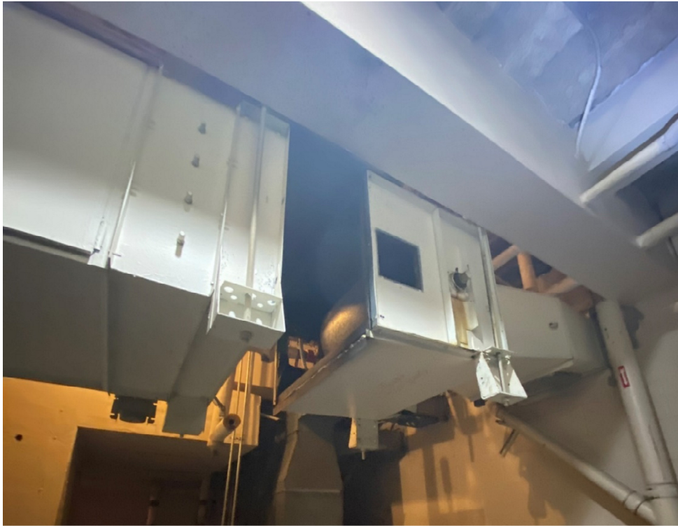
Figure 4 Air Handler tag AH-1. Note the missing section of the unit.
