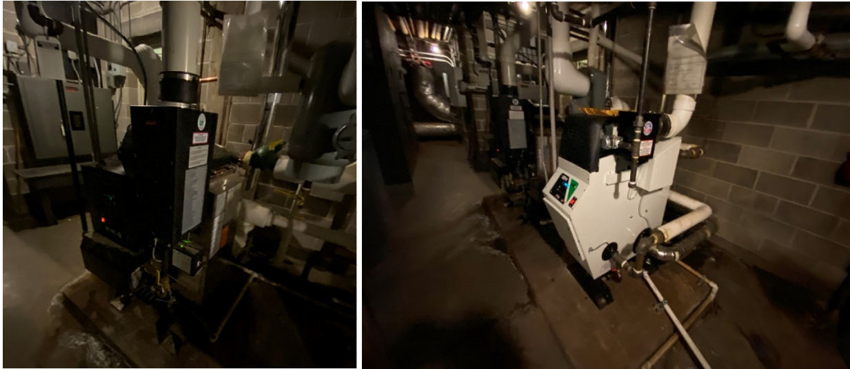
Figure 10 Bank building boilers.
