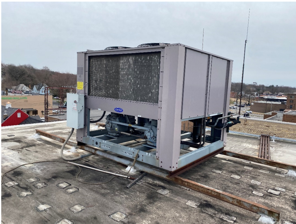
Figure 9 Bank building chiller.
