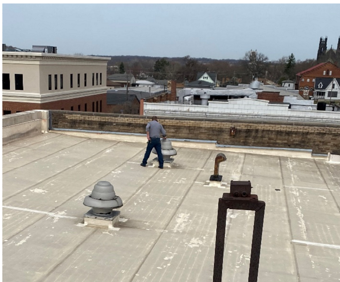
Figure 11 Bank building exhaust fans.
