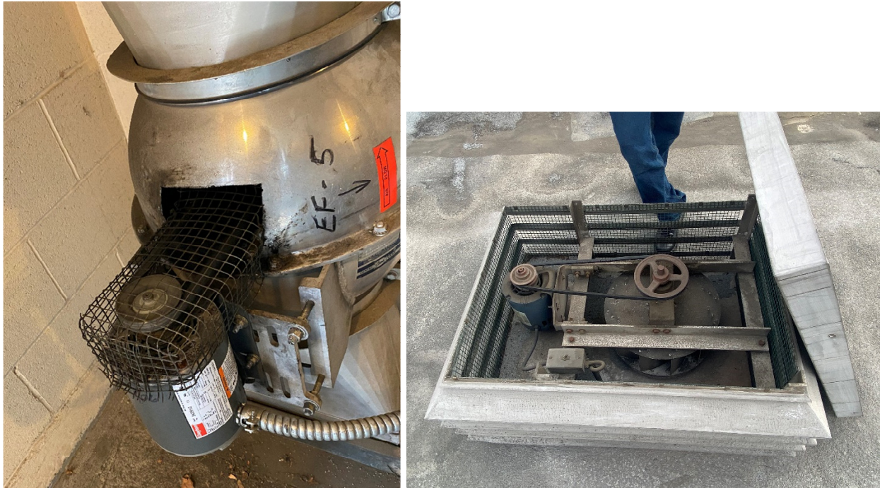
Figure 3 Exhaust fans. Note belt guard on EF-5 in the picture on the left.
