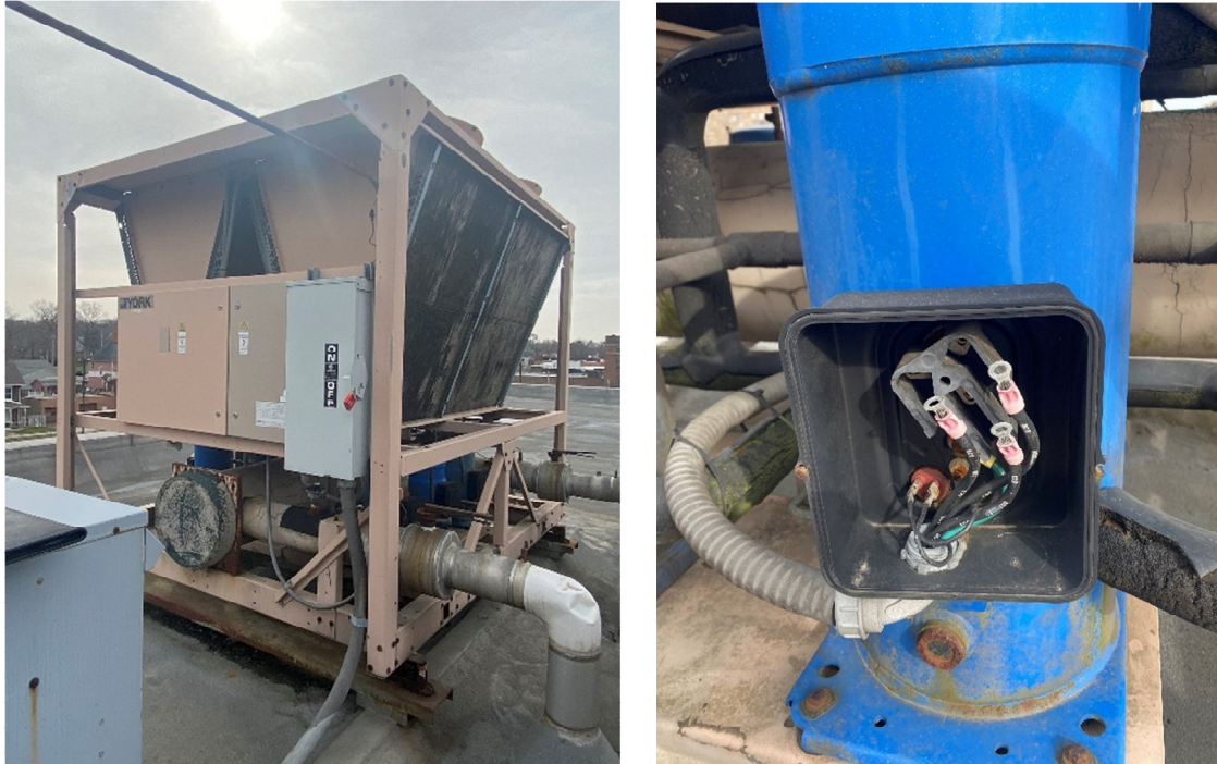
Figure 1 York Chiller on roof. Note damaged fins on coils. Second picture shows missing electrical cover and disconnected compressor.
