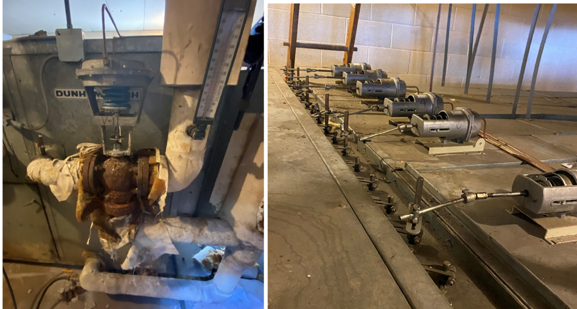
Figure 6 Control valve and zone actuators. Note disconnected actuator – second from right.
