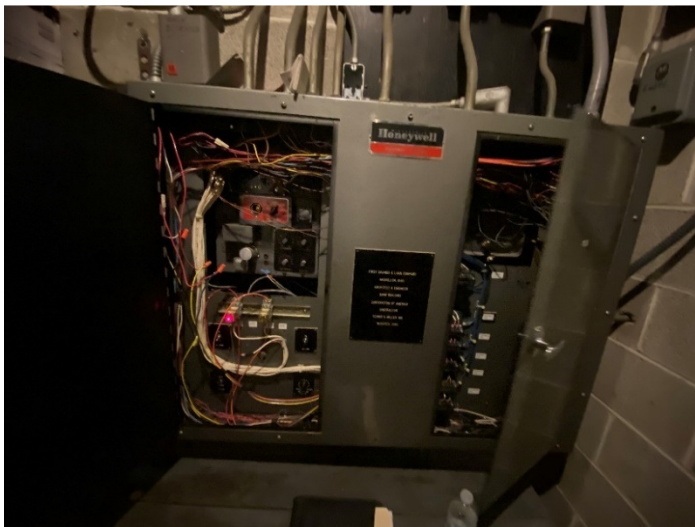
Figure 11 Bank building temperature control panel.
