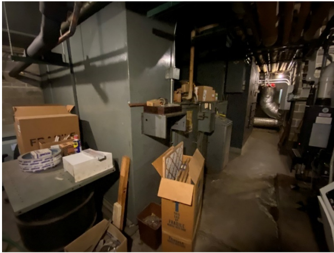
Figure 11 Bank building main air handler.
