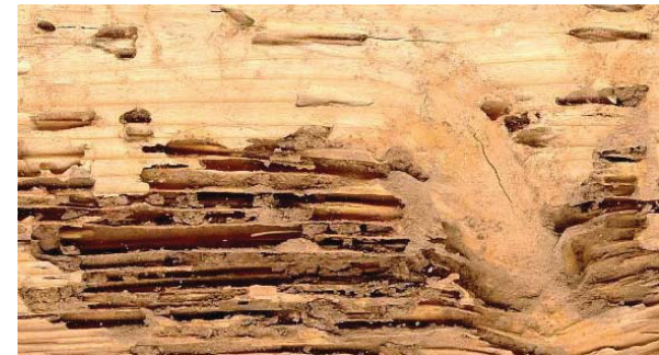
Galleries and debris in a wood floor joist indicate insect infestation.
