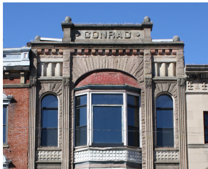
Sandstone cornice detail of the Conrad Block, 20 Lincoln Way East, c.1880s.
