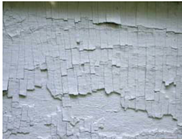
Alligatoring paint on exterior siding.
