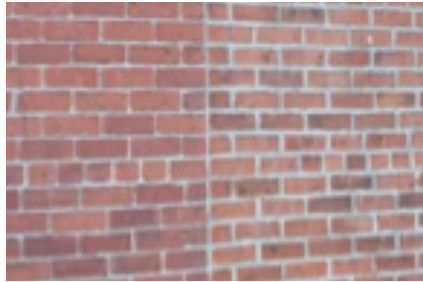
Exterior brick wall that has been built in two different time periods.
