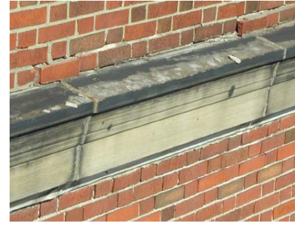
A loose stone cornice attached by metal fasteners indicate that its fasteners have failed.
