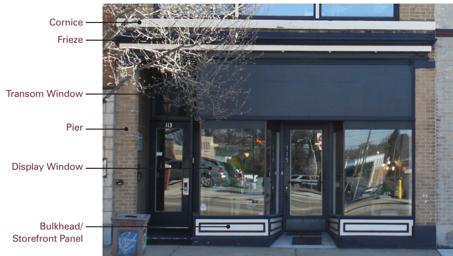
Components of a typical late 19th century commercial façade
