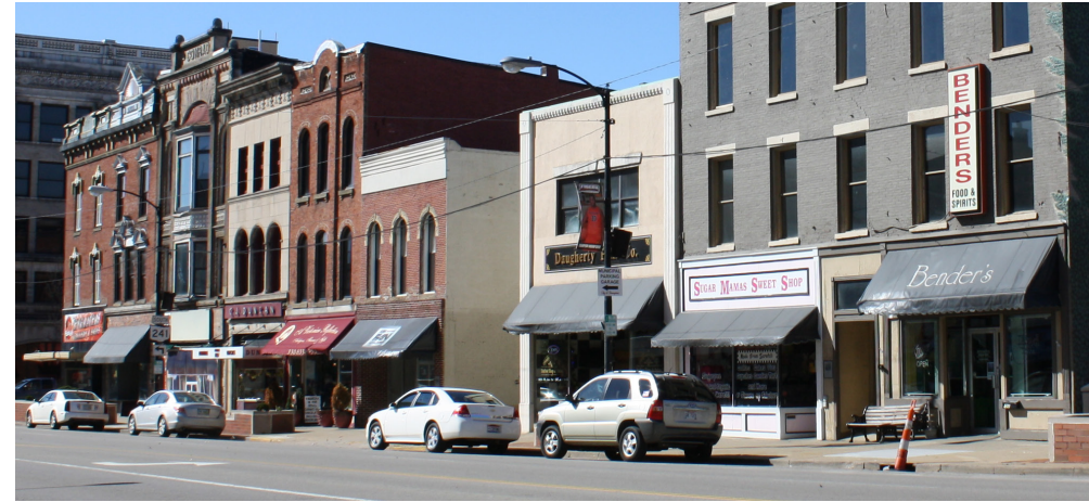
Existing awnings on commercial buildings lining Lincoln Way.
