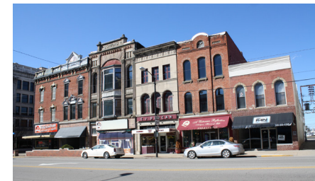
The simple design of the row of buildings on the northeast corner of Lincoln Way and Erie during the mid-19th century (upper, courtesy of the Massillon Museum) is contrasted with the same row of buildings today (lower). The upper facades (and storefronts) were completely transformed during the 1870s and 1880s in the more exuberant styles of the period, adding cornices, hoodmolds and a variety of windows.
