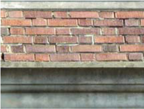
Deteriorating mortar and open mortar joints in a masonry wall.
