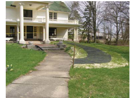
Grass pavers create a ramp without concrete and without altering the historic entrance to the building.
