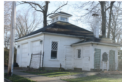
Example of an outbuilding in Massillon.
