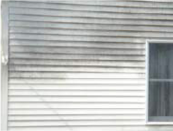
Mildew on painted exterior siding.
