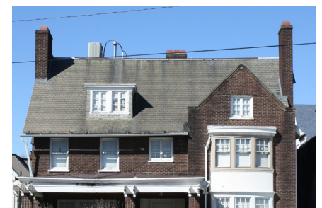
Gabled slate roof, chimneys, and dormer window of a residence along Lincoln Way E between 3rd Street NE and 4th Street NE.
