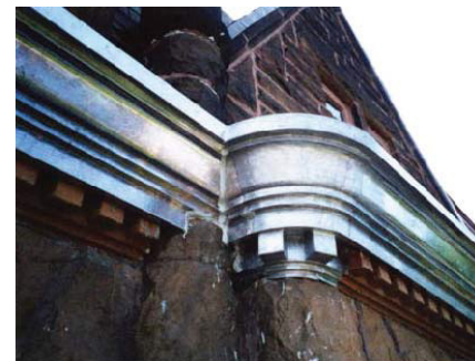
Missing elements are replaced with material to match and look like the original.
