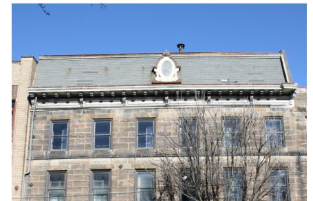
Mansard roof on a commercial building along Erie Street S between Charles Avenue SE and Tremont Avenue SE.
