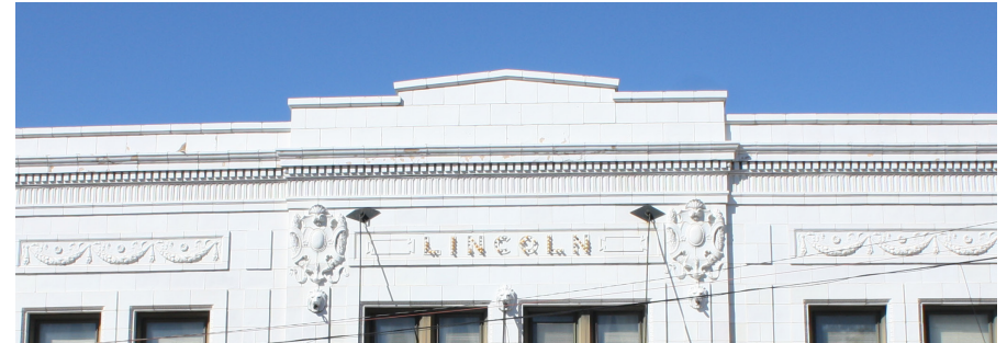
Terra cotta facing and ornamentation accents the facade of the Lincoln Theatre, built 1925.
