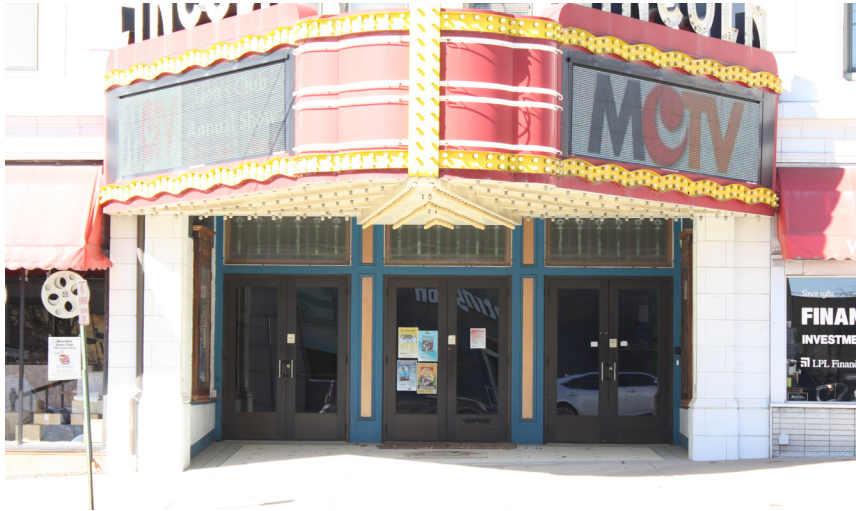
These double-leafed doors at the Lincoln Theatre are contemporary replacements with full-glass panels.
