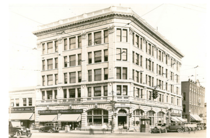
Photos show the McClymonds Building under construction, with a part of its facade in place, and as completed. The building, finished in 1910, is an excellent Classical Revival addition to the downtown. Courtesy of the Massillon Museum.
