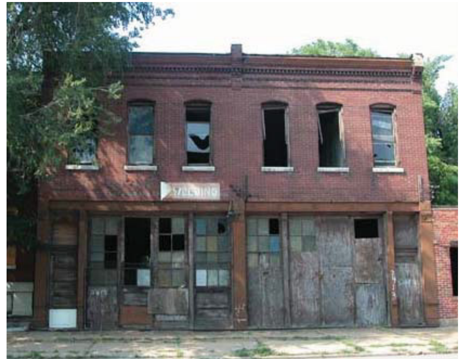
Lack of minimum maintenance over an extended period may render a building beyond rehabilitation.
