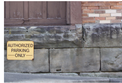
Exposed stone foundation of McLain Grocery Co., c. 1895
