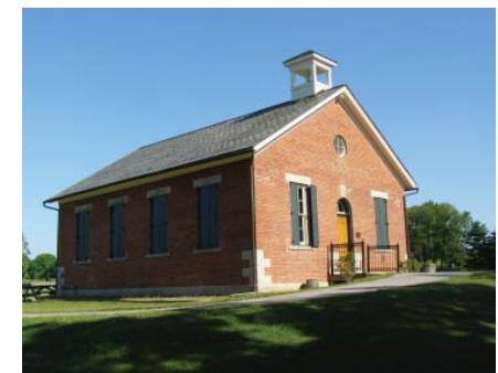
Land was graded and a sloped sidewalk installed to create a gentle ramp that makes the building accessible without destroying the appearance.
