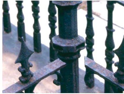
A corroded metal fence has failed at connections between the railings and the post.
