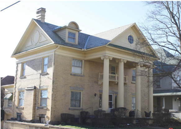
Top: Vernacular style with Queen Anne elements; Below: Neoclassical style, located in the neighboring Fourth Street National Register Historic District; see page 18 for a discussion about this style; Right: Queen Anne style
