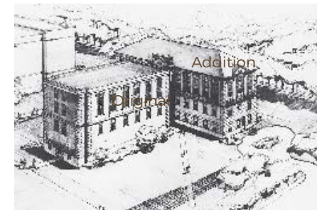
Example of a well-designed addition to the rear of an existing structure
