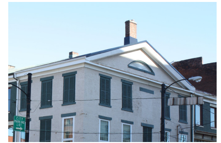
Gabled roof on a commercial building at the corner of Lincoln Way W and Erie Street S.
