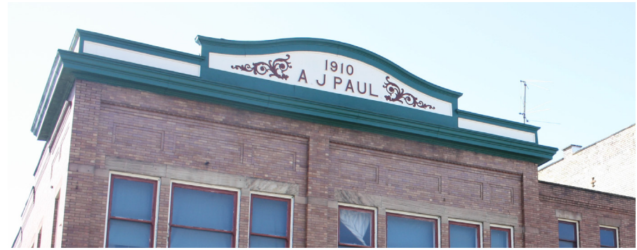
A wood parapet on the A.J. Paul Building, 109-13 North Erie Street.
