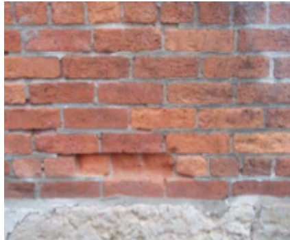
Exterior brick wall that has spalling due to water infiltration and improper repairs.
