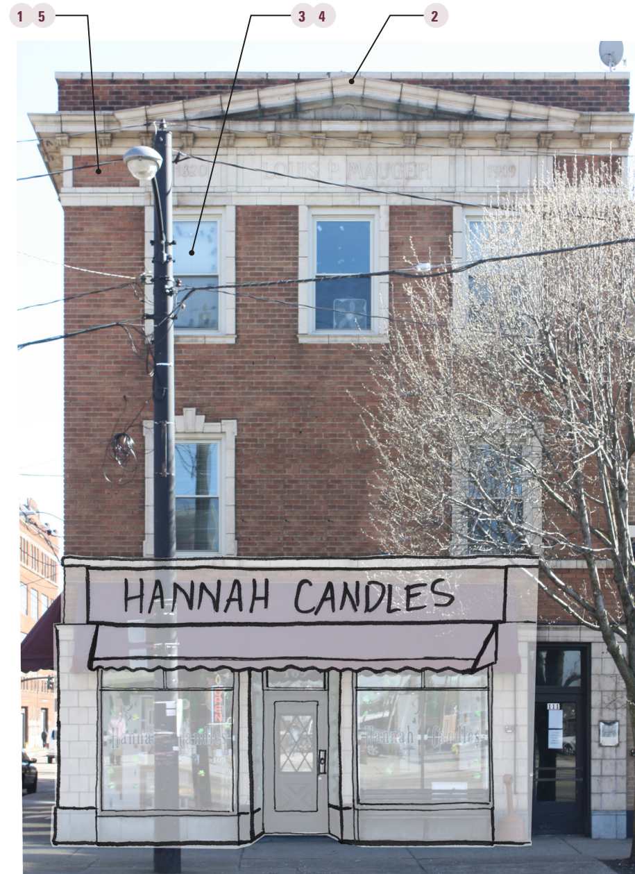
Neo-classical style, commercial example: Louis P. Mauger Building, 1919.
