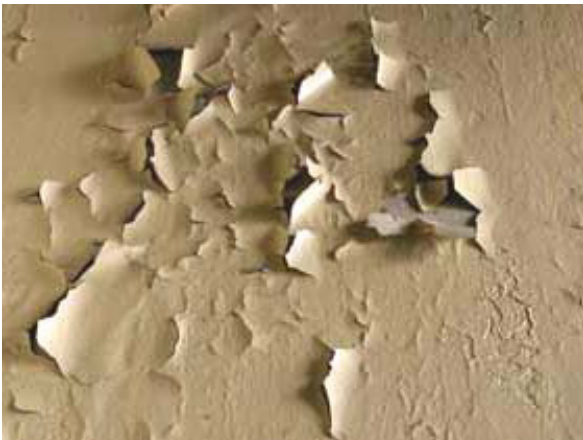
Peeling paint on interior wall.
