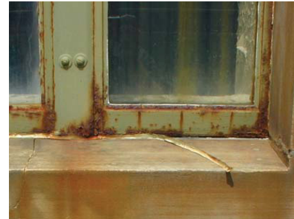
Corrosion/rust on a metal window sash resulting from exposure to moisture and air.
