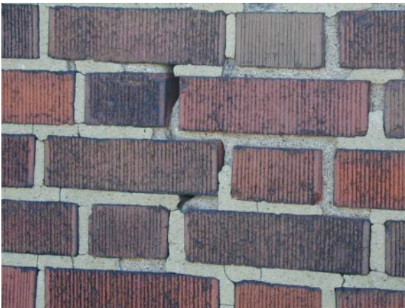
Previous poor repointing. Repointing mortar is falling out of joint due to improper execution.
