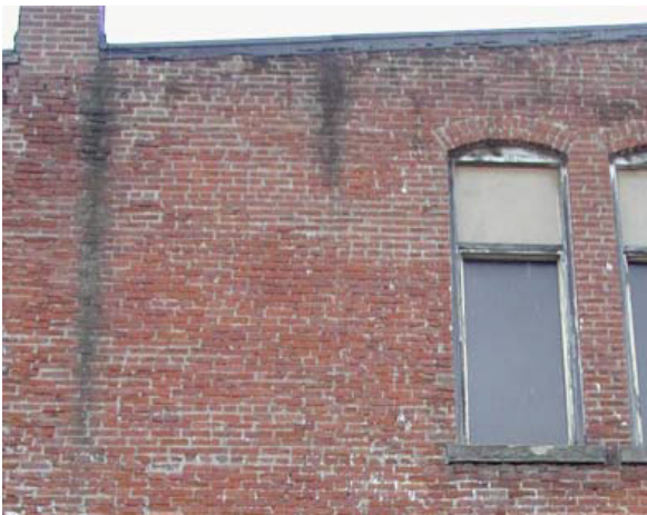
Dirt and stains on brick caused by runoff from the roof and corroded metal coping.
