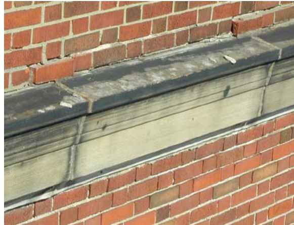
Loose brick falling out of wall due to poor conditions of mortar joints (moisture and movement in masonry system).
