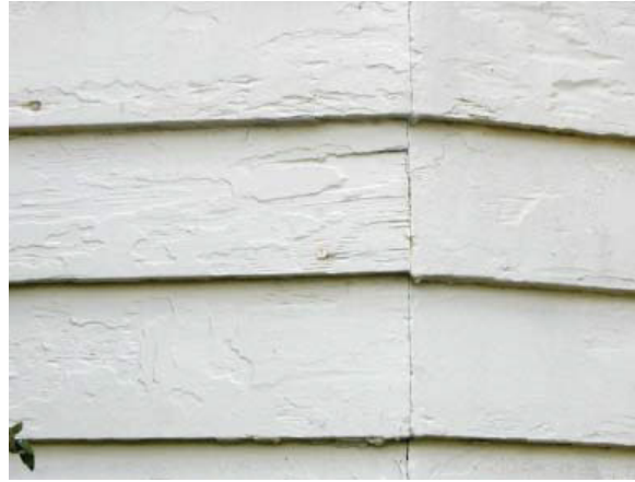
Improper preparation before applying paint results in a poor finish.
