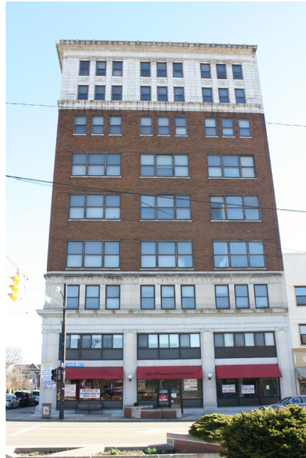
The upper facade of the Ideal Department Store Building, built 1918, has large areas of window in relation to wall surfaces.
