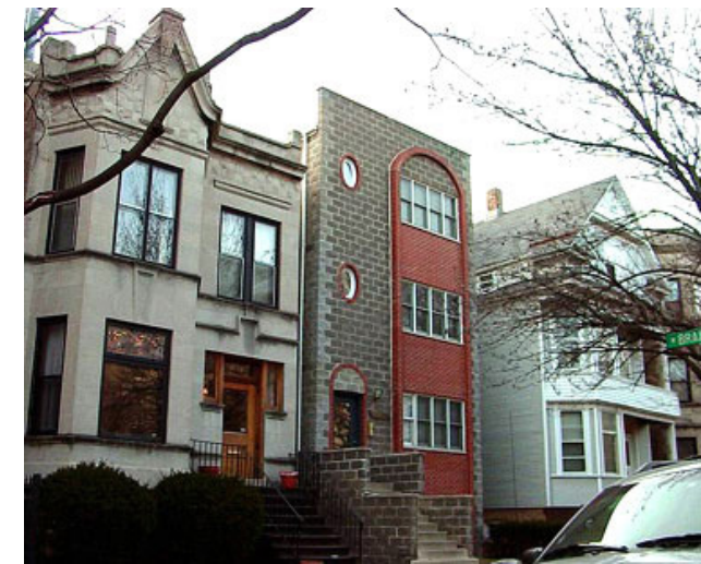
Example of an infill that poorly relates to adjacent existing structures
