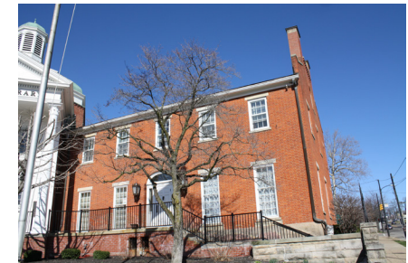
Top: The James A. Vaughn House, 122 Broad Blvd., has been converted to office use.
