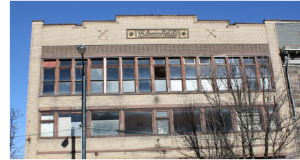
Windows create important visual patterns in the upper facades of downtown buildings, such as Bloomfield's on Erie Street between Charles Avenue SE and Tremont Avenue SE.
