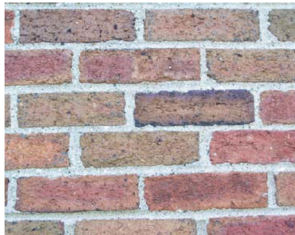
Damage to brick caused by sandblasting.
