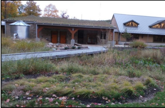
Large cistern (silver tank) capturing stormwater runoff from a green roof at the Cleveland Metroparks West Creek Reservation Watershed Stewardship Center. Credit: Northeast Ohio Regional Sewer District.
